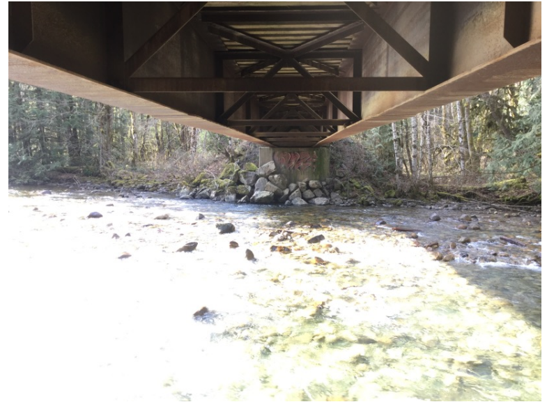
Left Bank Abutment when facing downstream
