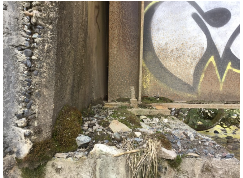
Upstream left bank bearing bolt
