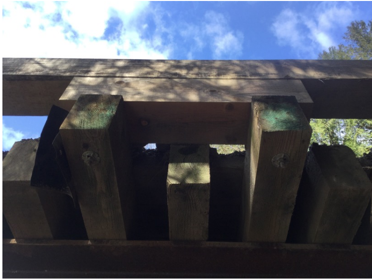
Timber risers span 3 ties
