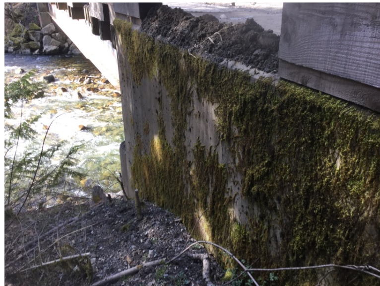
Upstream right bank wing wall
