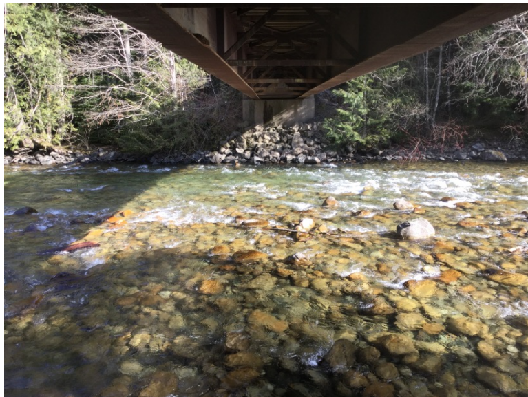
Right Bank Abutment when facing downstream
