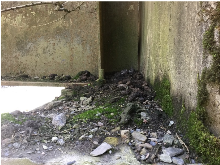
Downstream left bank bearing bolts
