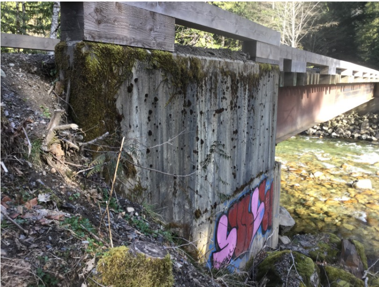
Upstream left bank wing wall
